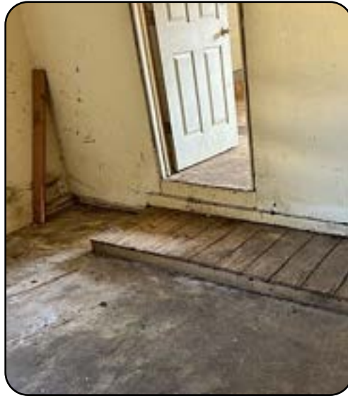
Floors at different levels downstairs would need to be raised or lowered to be ADA compliant. New flooring would be needed throughout.
