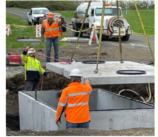
Holding Tank Install @ South Side Park
