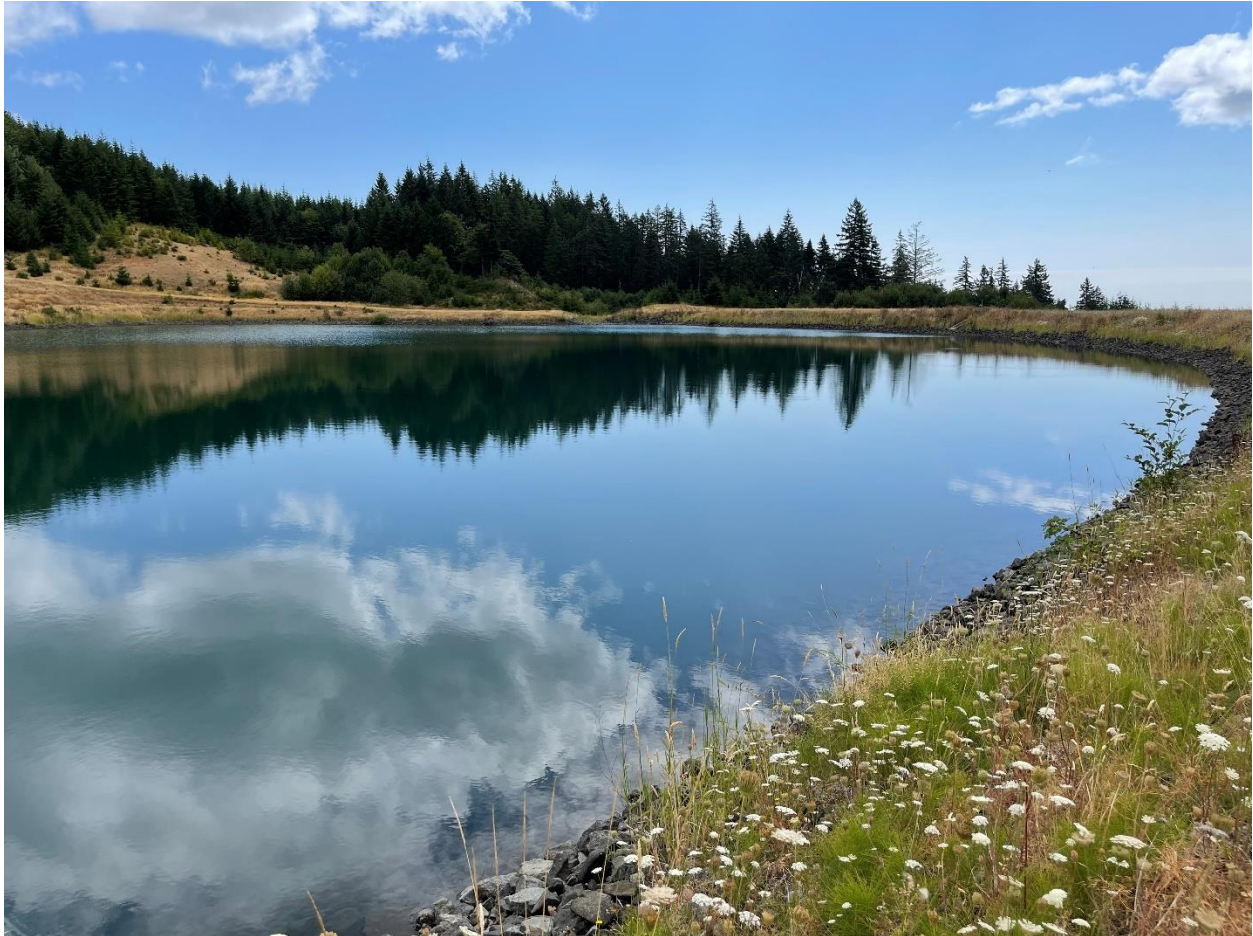
Stoney Mountain Reservoir
